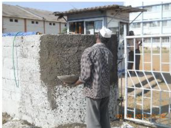
During the external Crush sand & River sand plastering
