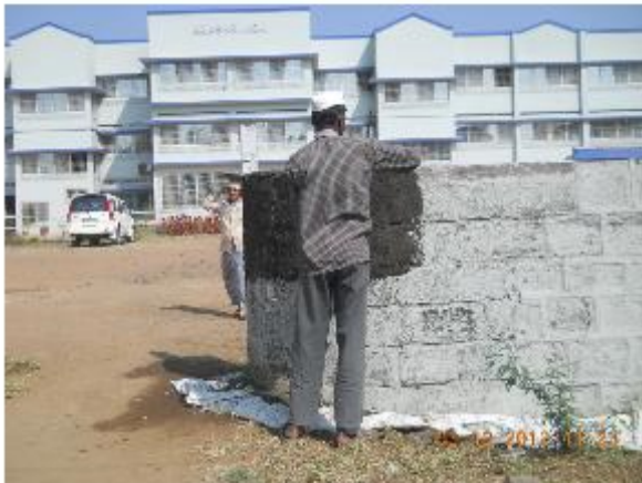
During the external Crush sand & River sand plastering
